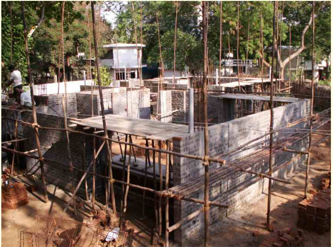
The new building is rapidly coming up !
